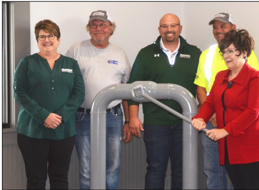
IEDA Director Debi Durham turns the ceremonial valve signifying completion of the new gas line expansion by Manning Municipal Utilities. Shown, from left, gas department staff Carla Hacker, Dick Mundt, MMU General Manager Jeremy Carroll, Denny Steffes and Durham.
